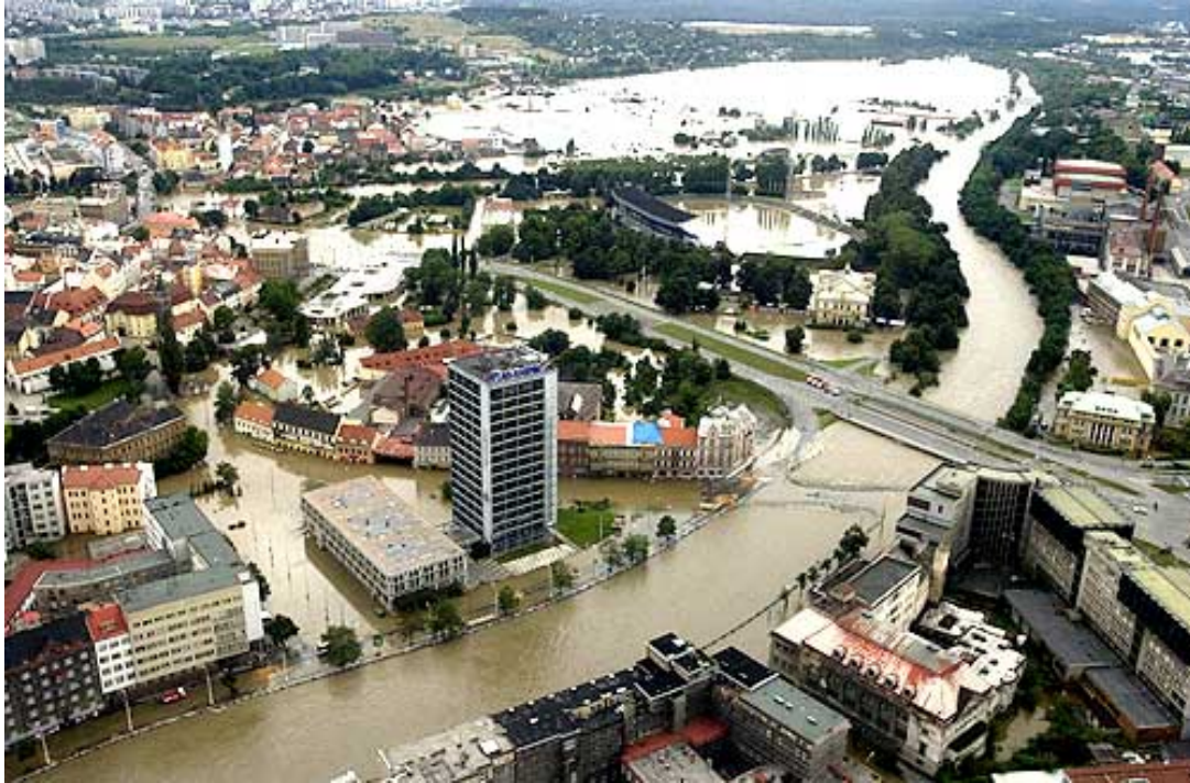
Figure 3.2: Prague 2002: overview of flooded city (ANSA, 2002; in www.corriere.it )
